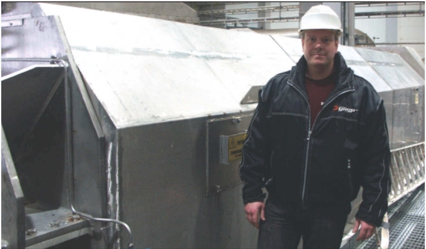
Anders Dahlberg by the screw press that now runs better and with a reduction of the energy use.
